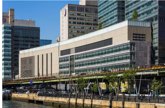
NYU Langone Energy Building, © Jeff Goldberg / Esto
