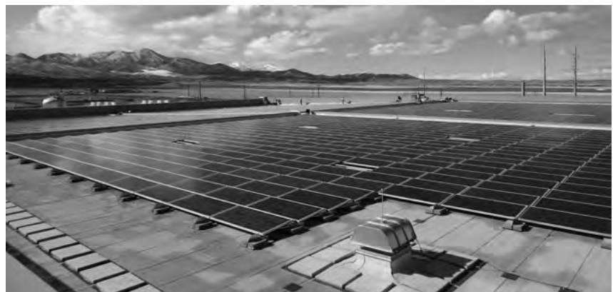
➡ The roof of eBay’s Topaz data center in South Jordan, Utah.
