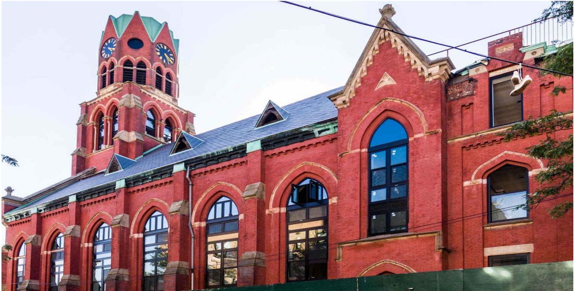
St. Marks Evangelical Lutheran Church in Bushwick neighborhood in Brooklyn, New York build 20 affordable units right into their old church structure.
